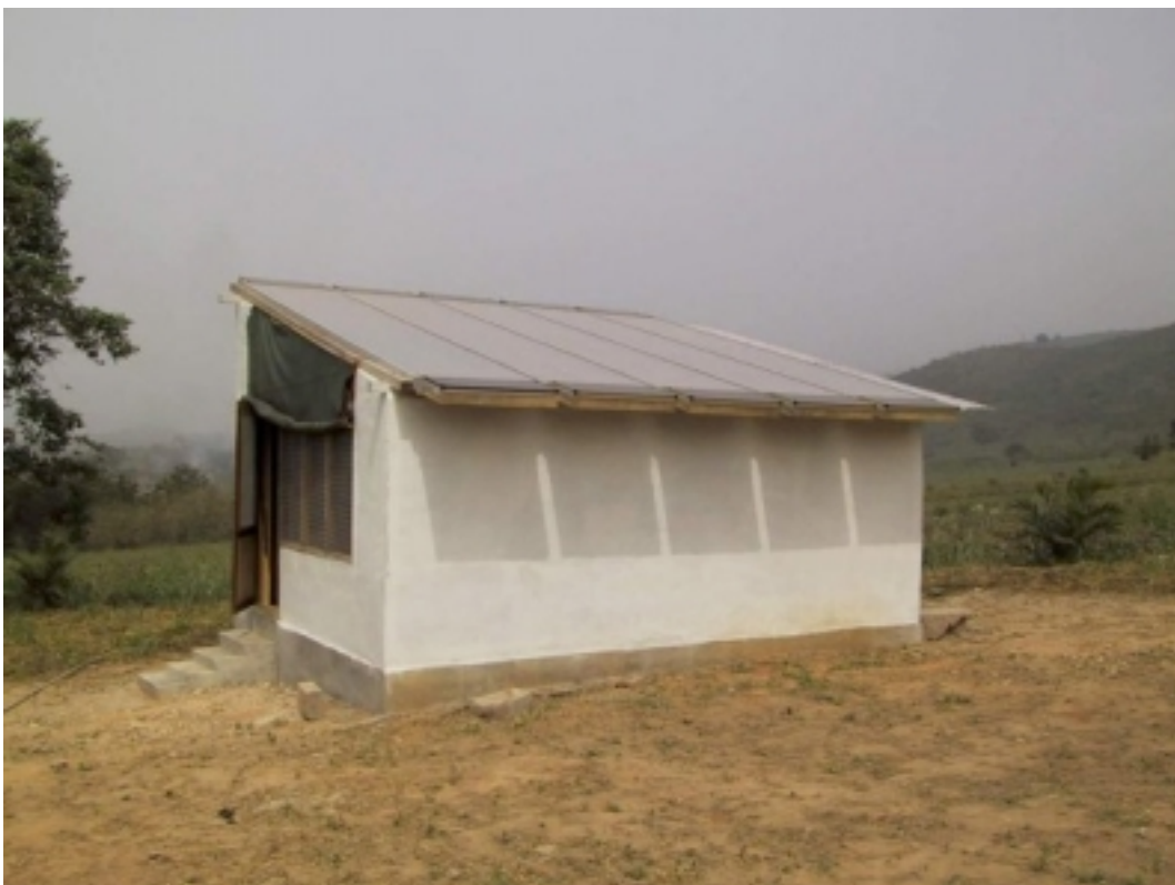
Figure 6.1. The solar crop dryer seen from the south.
